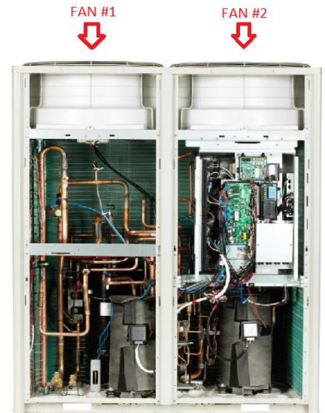
Fan #1 is on the left-hand side of unit
