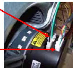
TECMate 16-pin Connector
